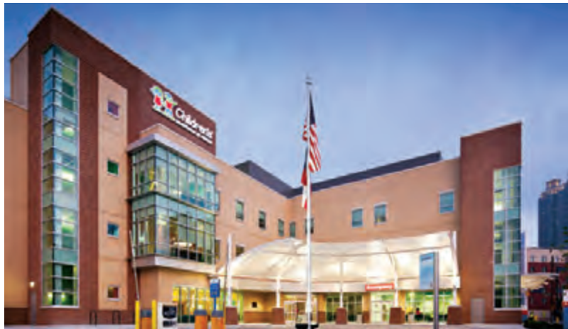
THE NEW ENVIRONMENTALLY FRIENDLY HUGHES SPALDING BUILDING WAS DESIGNED WITH PEDIATRIC PATIENTS IN MIND.
